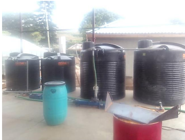
Figure 6: Protein and whey collection tanks at small-scale green biorefinery in Uganda
