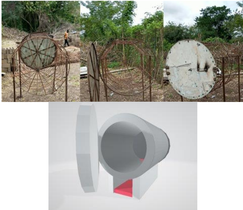
Figure 10: New furnace build at INP-HB with metallic skeleton and bricks
